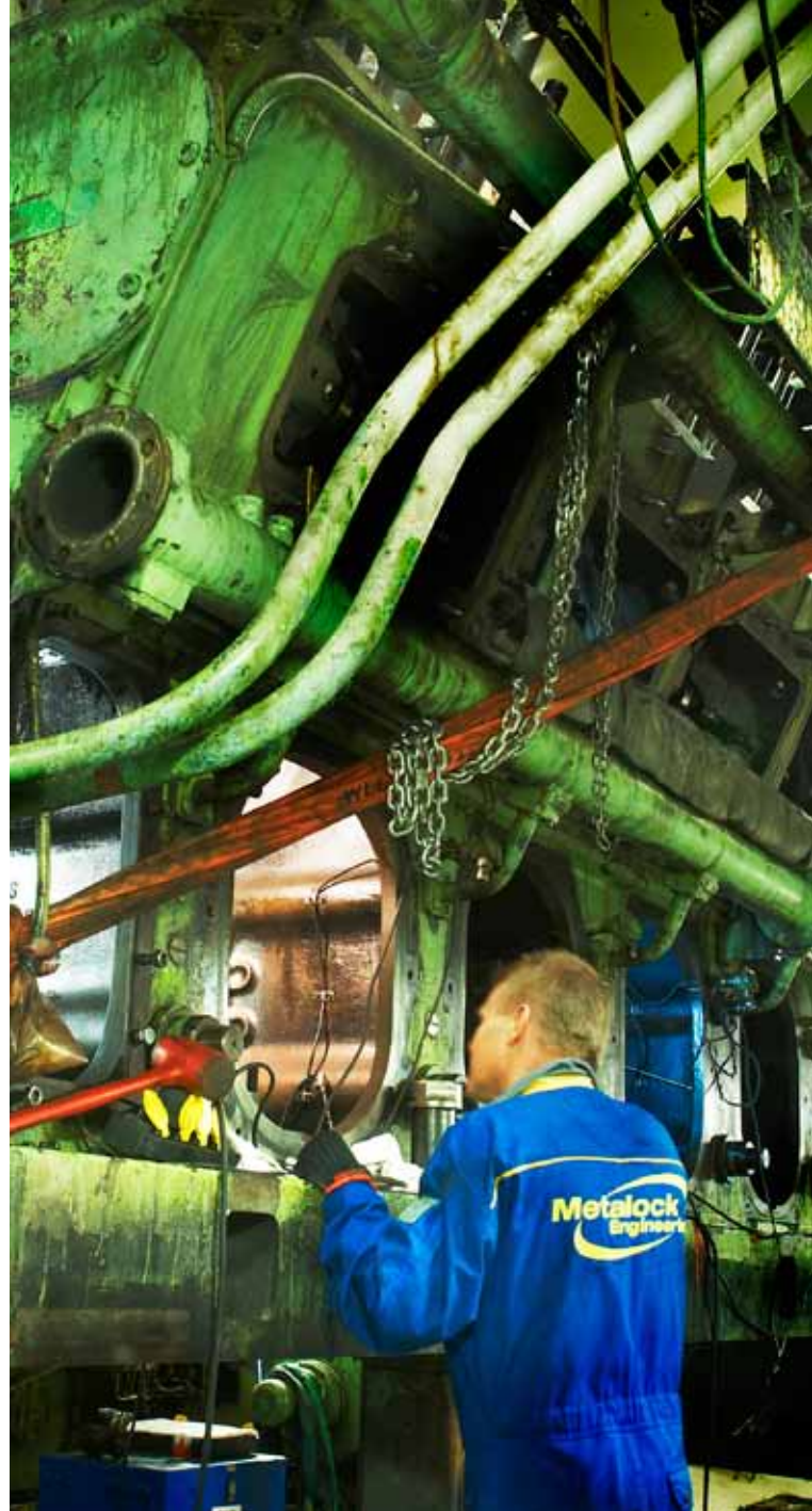
Mobile drilling of main engine, M/F Stena Danica
